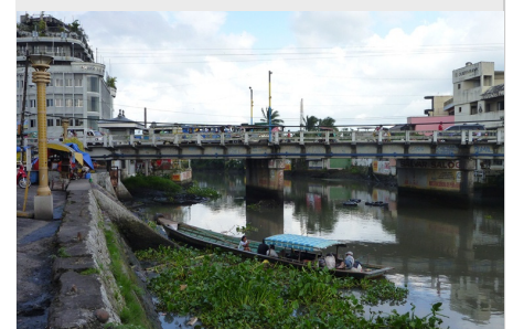
River environment— Poor water quality due to outlet of untreated sewerage
